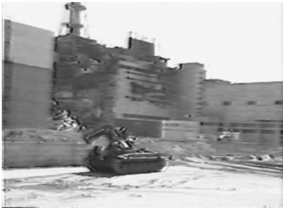
Fig. 31 - Roof hole following explosion in Unit 4
