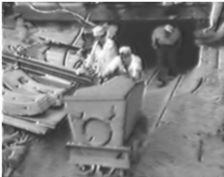
Fig. 36 - Excavating the tunnel beneath the reactor building
