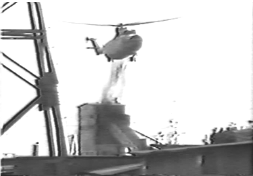
Fig. 33 - Shielding being air-dropped onto the reactor core
